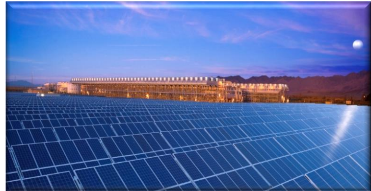
Stillwater Solar PV
